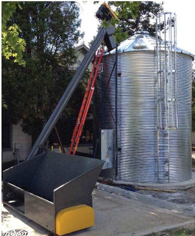
A receiving bin and feed auger fill a 15-foot diameter storage silo adjacent to the boiler room
